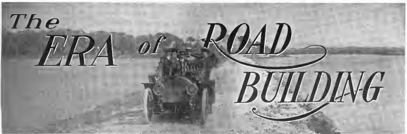
THE CAUSEWAY ACROSS ROSE BAY ON THE FLORIDA EAST COAST MOTOR HIGHWAY.
